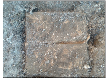
Stones that were part of the original foundation.
