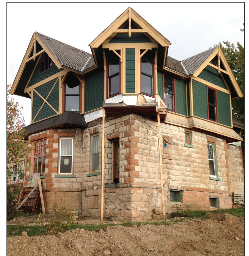
Work will soon begin to restore the house's original front entrance.
